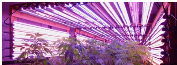
T5HO Installation in a California Greenhouse (Photo courtesy of Marigold Lighting)
